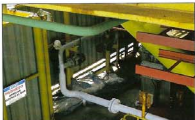
Nansulate is seen here applied in a high heat application.
